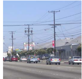
ROSECRANS BEFORE UNDERGROUNDING
